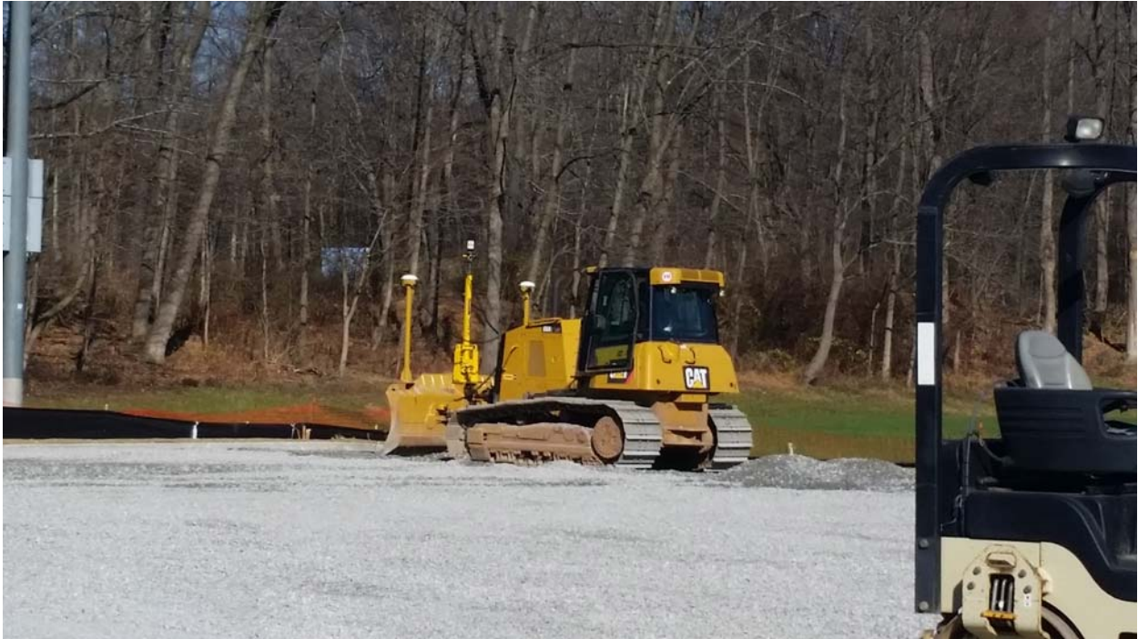
Figure 6: Final grading of finish stone.
