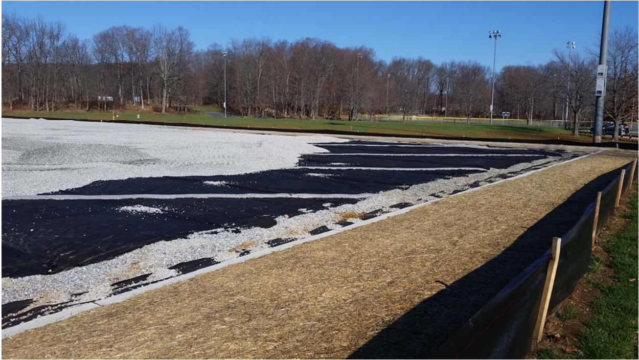
Figure 4: Curbing and perimeter drains complete, installation of drain stone beginning.
