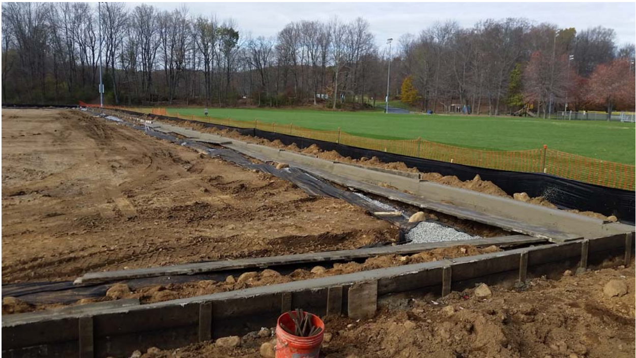
Figure 3: Perimeter drainpipe and curbing installation
