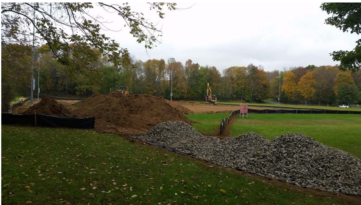
Figure 1: Stripping of topsoil\rough grading
