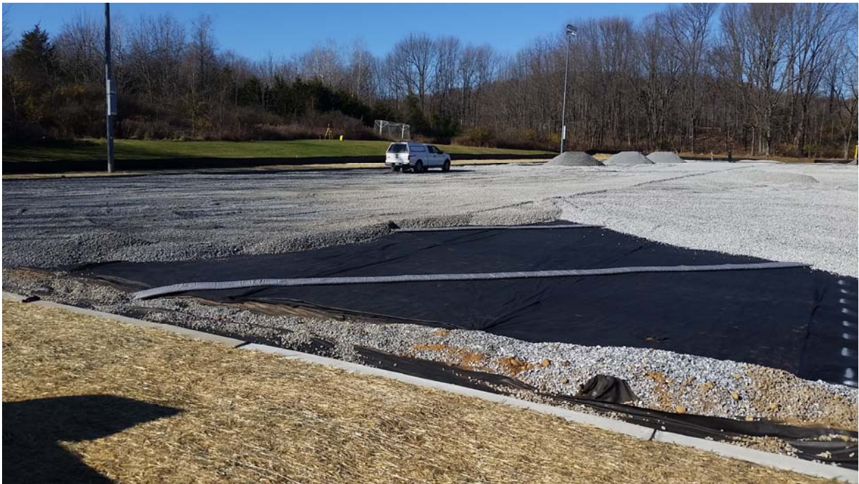
Figure 5: Drain stone installation
