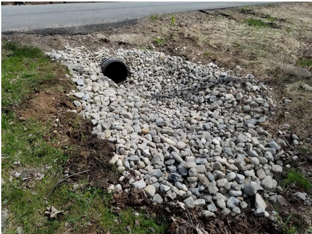
Figure 7: Outfall of Drainage Pipe Crossing Edison Road
