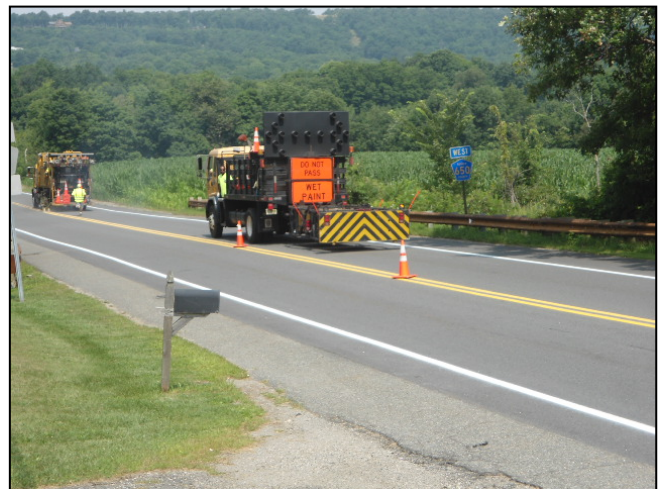
Typical Striping Operation
